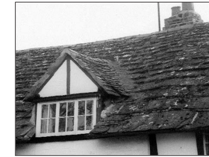
Horsham Stone Roof
