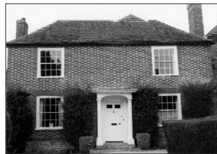
In contrast, are the larger scale brick built Georgian and Victorian buildings. Many of these are built over timber framed cottages.
