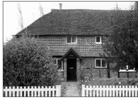
The timber framed buildings are often infilled with plaster or brick nogging, some with tile hanging on the upper storey.
