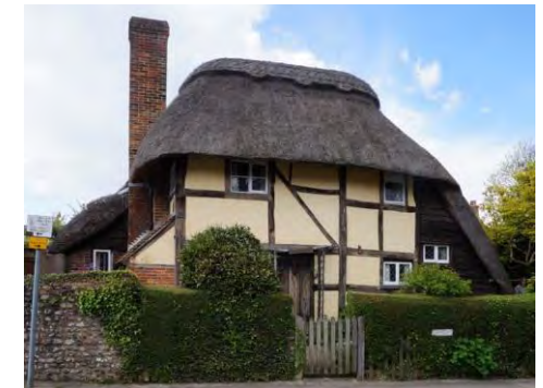
'Saxon Cottage' on Church Street.
