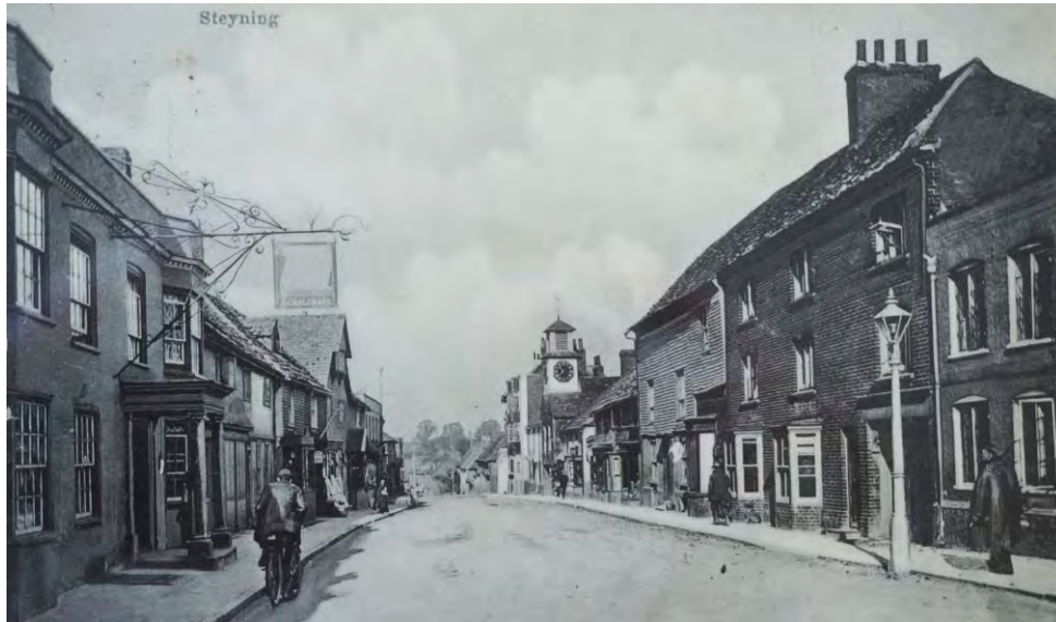
High Street, looking north
