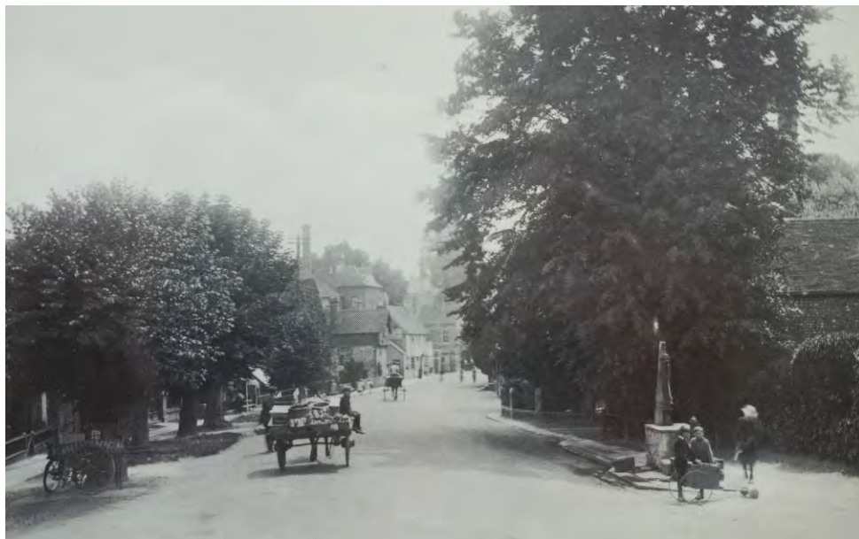
High Street, looking south
