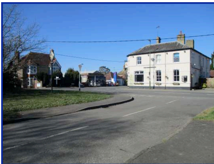
Figure 6: The Partridge Pub & Pretty's Garage Junction of High Street & Church Road
