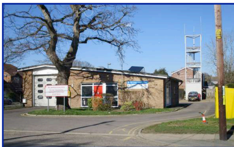
Figure 5: Fire Station, Partridge Green
