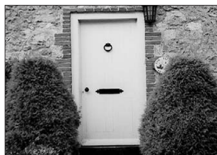
Doors are generally simple wooden designs, some with glazing and often with steps leading up to them.
