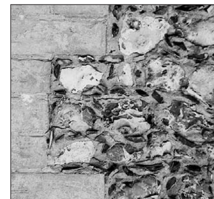
Flint galleting (chips of flint in the mortar), Vine House, Church Street.
