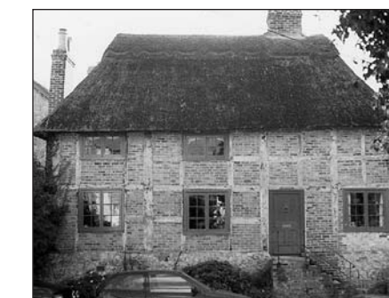
Timber frame buildings, Panel Cottage.
