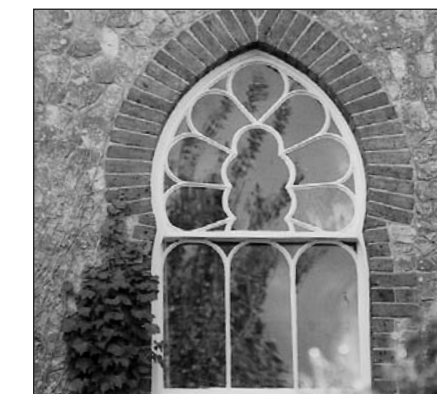
Cast iron gothic windows, the Manse and Chapel (Pottery).
