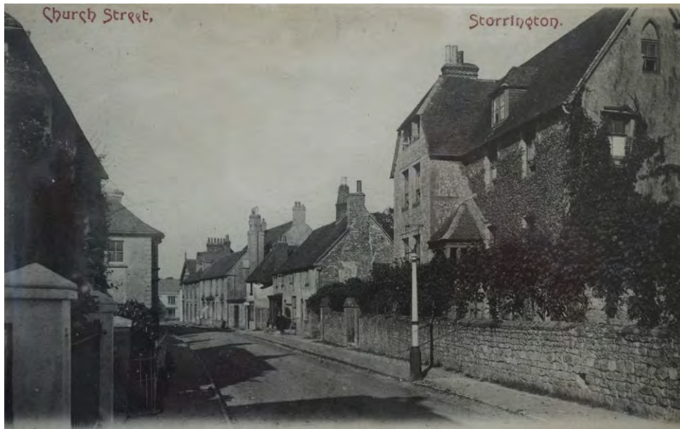
Church Street, looking north.
