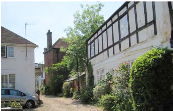
Brewers Yard, looking towards High Street.
