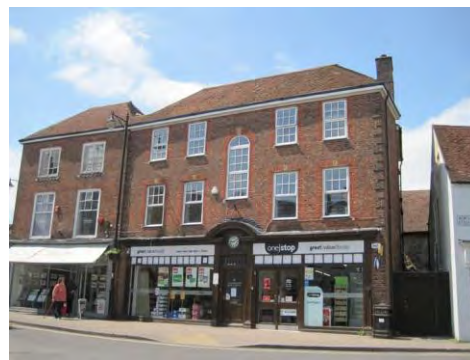
1920s post-office building - a sensitive development.
