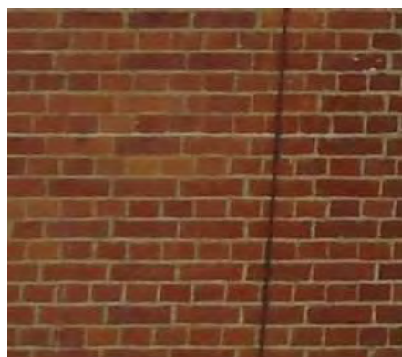
English bond with alternate rows of headers and stretchers
