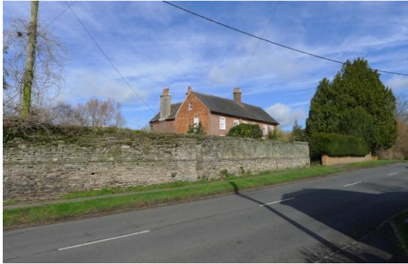
Stone boundary wall at north end of the High Street.
