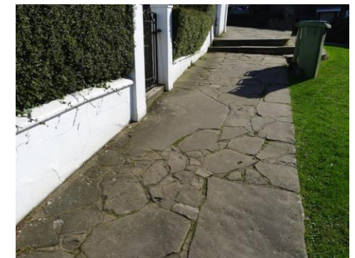
Historic natural stone paving.
