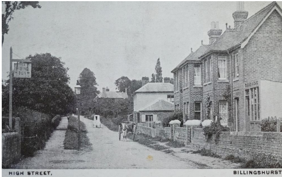
High Street, looking north
