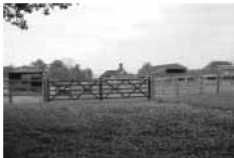
New gateway of appropriate construction
