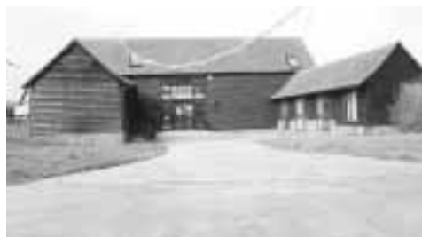
Barn conversion to commercial use
