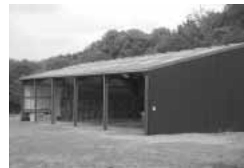
Modern barn construction
