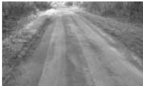
Widened country lane
