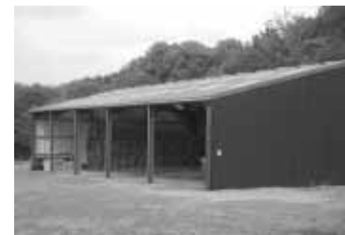
Modern barn construction
