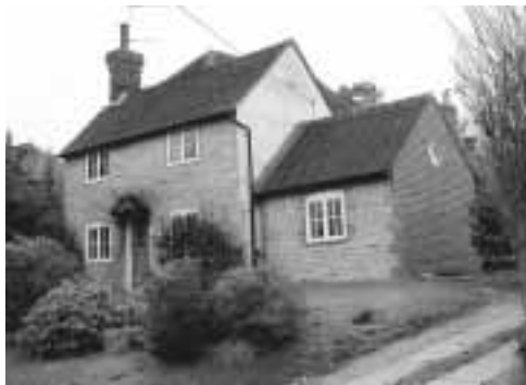
Sensitive extension to cottage in Friday Street
