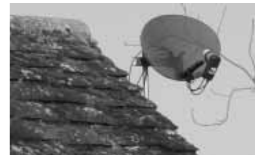
Satellite dishes in juxtaposition with Horsham stone roofing
