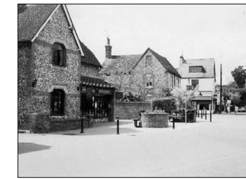
The realigned road, pavements, car park and side road alongside Bramber Villa create an open feature
