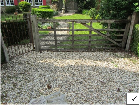
A shingle drive (porous)
