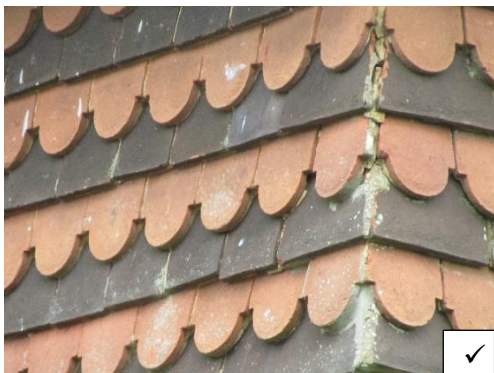
Two colour tile-hung wall
