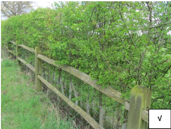
A green living hedge with post and rail and wire mesh fence
