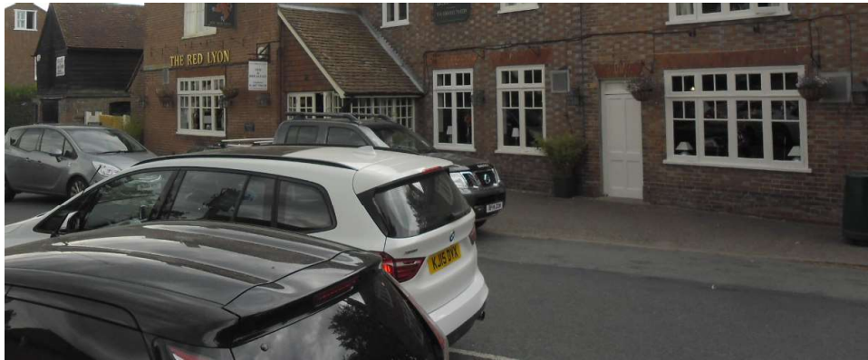
Parking and use of less sensitive surfacing detract from the Conservation Area
