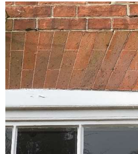
Decorative headers above the windows
