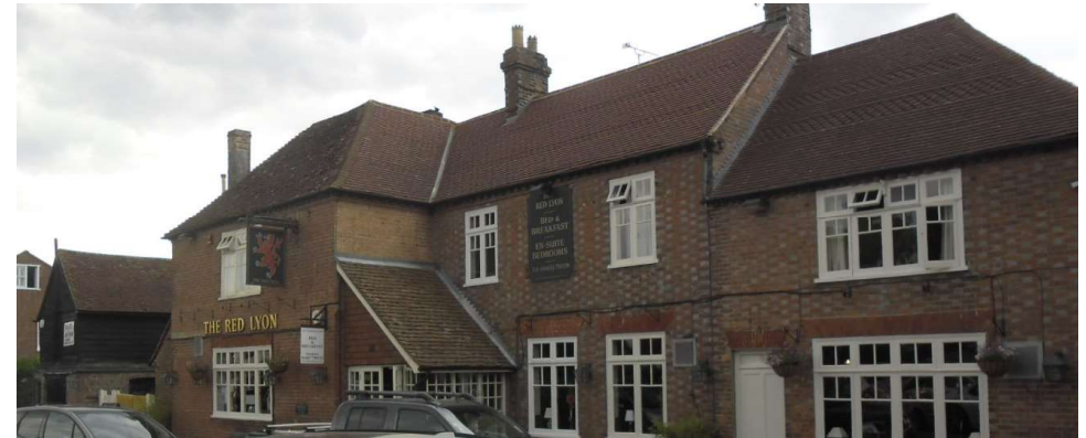
The Red Lyon forms a prominent building in the streetscene, which is read in context with the Old Post Office, shop and bakery on the opposite side of The Street
