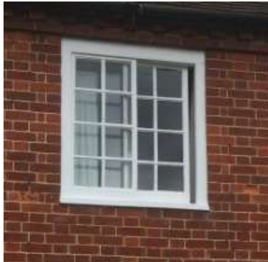
Horizontal sliding sash window also known as Yorkshire sliding sash
