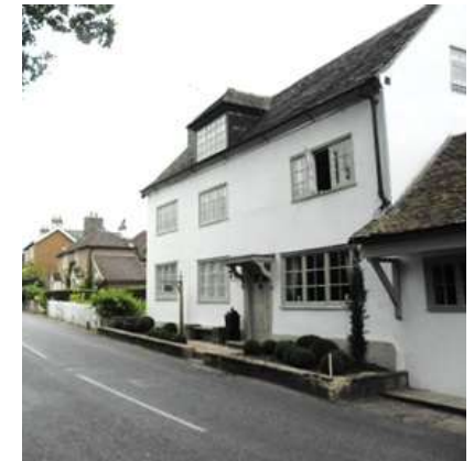
Starr Inn House – reinstatement of the porch and door taking inspiration from its historic predecessor. Details were inferred from old photos, and based on research and an understanding of the building rather than a possible interpretation.
