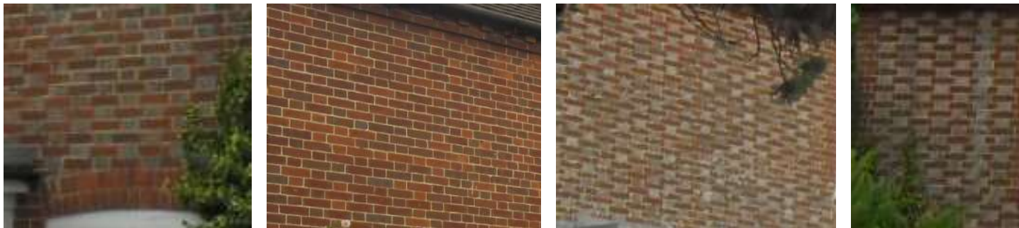
Examples of Flemish bond brick work within the conservation area. Many properties exhibit bricks with a dark header and a red stretcher creating a pleasing, characterful appearance
