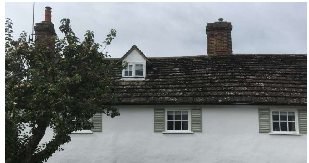
Horsham Stone slate roof
