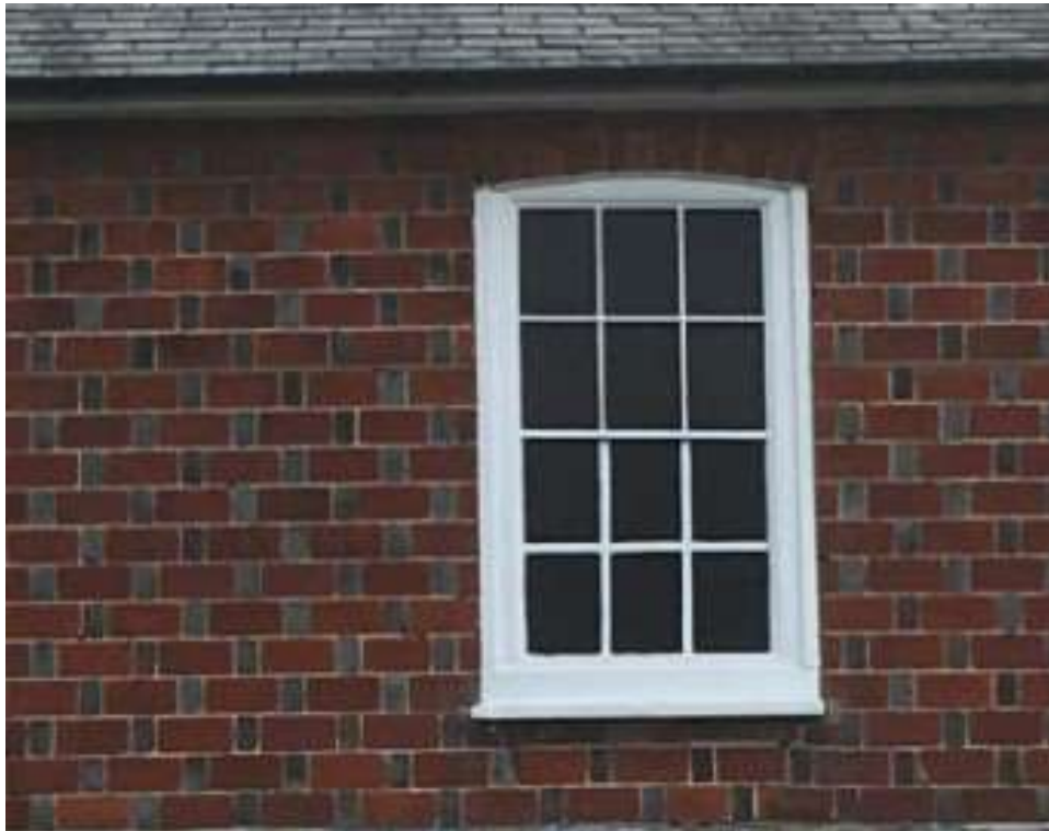
Rat trap brick bond, with the bricks placed in a vertical position, which creates a cavity within the wall
