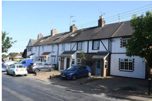
The cottages in East Street, another important aspect of village architecture
