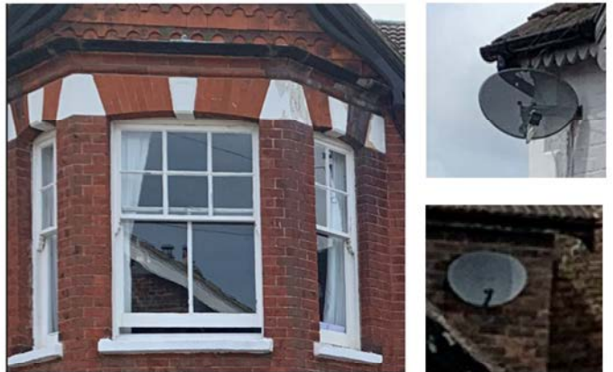
Timber sliding sash windows and satellite dishes with examples in a prominent and less prominent locations
