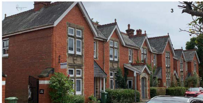
Images 3 - 1 - 4 Peel House and Bailey House, Bartelot Road "Former police station buildings. Peel House is two storey with four gables fronting the road, and central porch and door. West Sussex County shield carved in stone between ground and first floor. Brick with stone dressings and a slate roof. Bailey House built to similar designs, however of a smaller street front with two gables. In use as a police station between 1894 and 1973. Now used as offices. Gates to rear yard display the Centenary 1994 police badge. Built 1884." Image 1 - Christian Life Church East Street "Previously the Pentecostal church and originally the Primitive Methodist church. Brick built, with 3 bays, the central one over the door below. Decorative terracotta panels with pediments and finials. Plaster decorative panels. c.1891." Image 2 - 51 and 53 East Street "51 East Street is a 2 and a half storey Victorian brick building, with projecting bay window at first floor and a quality traditional shop front at ground floor. It forms a group with number 53, of which the most prominent feature is the corner tower at first and second floor. c.1890" Text taken from the 2011 Horsham Town Local List.
