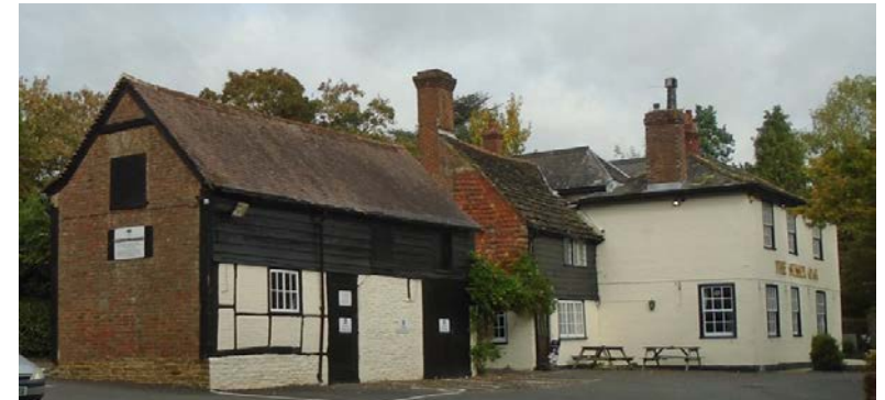
The Sussex Oak, with visible timber frame to the stables, and the timber frame of the oldest part of the public house clad in tile hanging, and weatherboard with brick infill. The buildings are roofed in clay tiles, slate and Horsham Stone slabs, with varying size chimney.
