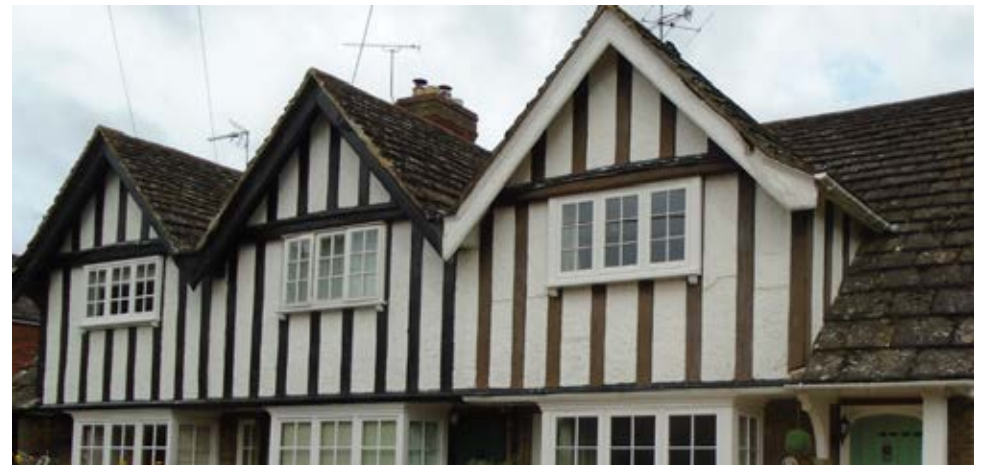
Horsham Stone slate roof
