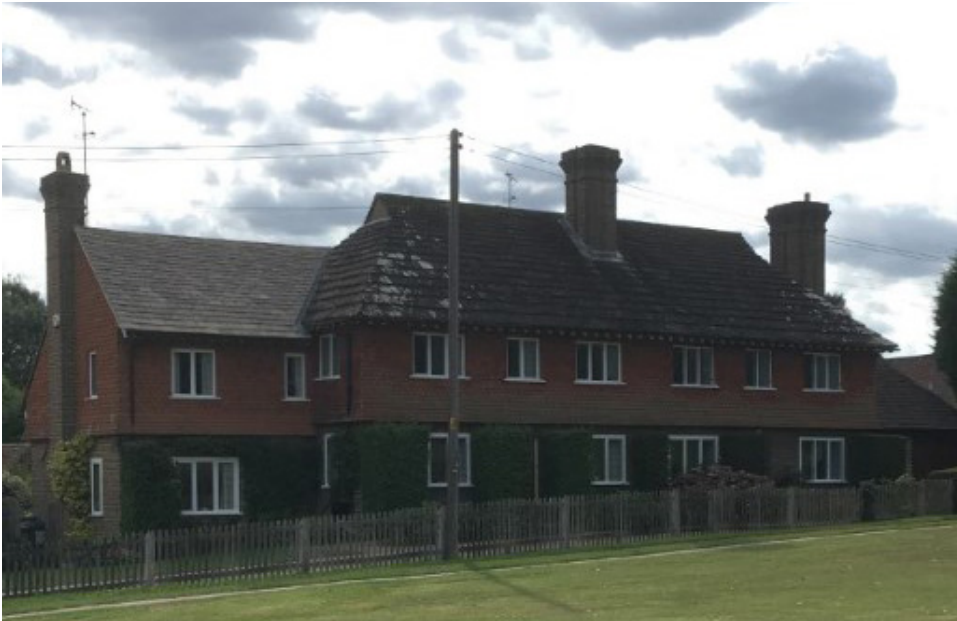
Traditional Horsham Stone slates on main roof with imitation slate to extension which do not have the same appearance as the original
