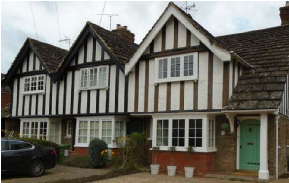
3, 5 and 7 Bell Road built in a vernacular revival style with Horsham Stone roofs and close studding to the first floor, and a symmetrical form
