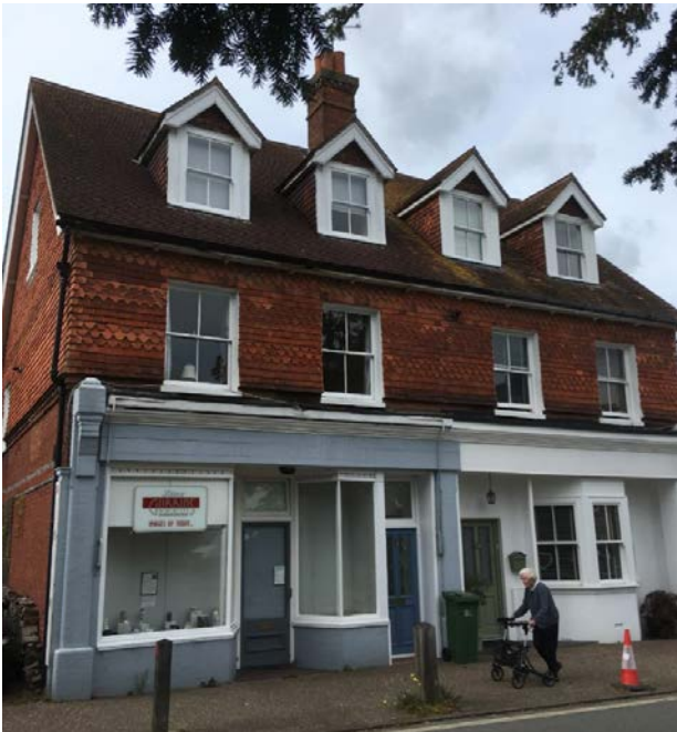
Chewton and Little Hammers have an exposed timber frame
