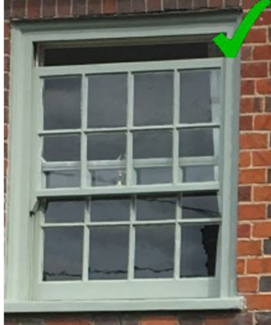
Photograph of a window with historic glass which creates a distinctive reflection and distortion
