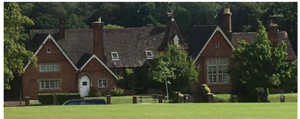
The former school built in 1878 by Sir Arthur Blomfield
