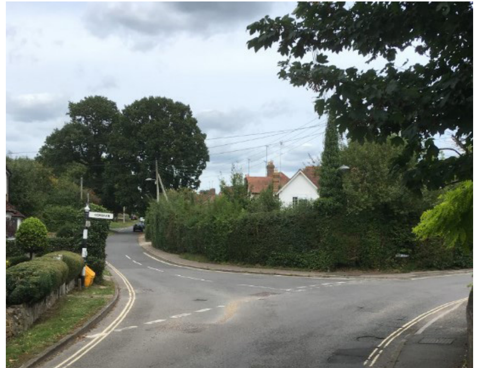
Junction of Tilletts Lane and Friday Street looking north east with the properties at the junction forming a soft introduction to the conservation area
