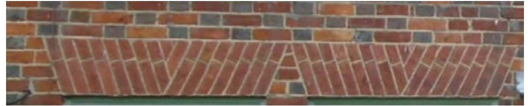
Decorative headers above the windows
