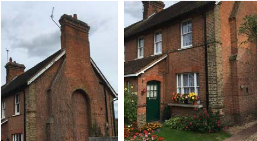
Detailing in terrace from 7 – 21 Church Street, with chimney details, porches and front gardens
