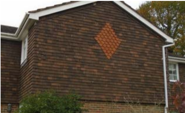
A lack of appropriate detailing and understanding of the architectural features have resulted in the terrace having an incongruous appearance
