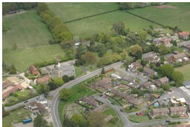
Fig.2: Aerial View of Lower Beeding
