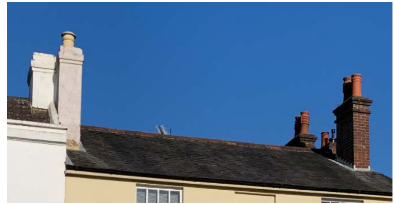
Variation of chimneys within the conservation area
