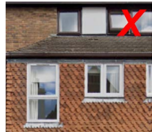
Positive and negative windows within the conservation area showing modern and historic sash windows.
