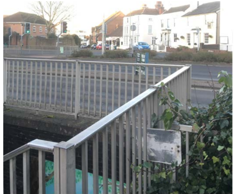
Pedestrian crossing and entrance to the underpass connecting London Road to the town centre and principal shopping area
