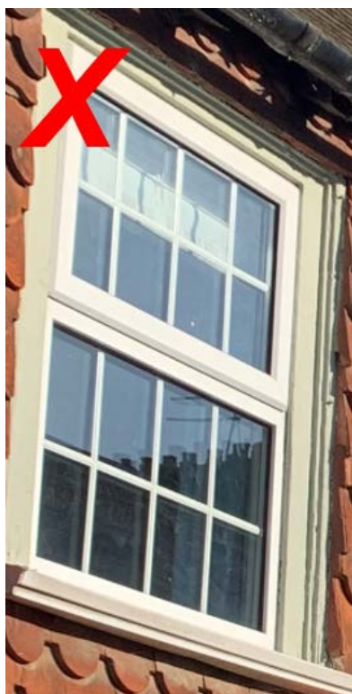
The use of plastic windows do not reflect the character of the conservation area, this is particularly evident in the lack of detailing and the changes to opening mechanisms.
