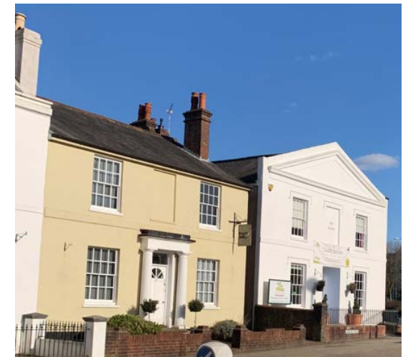
16 - 20 London Road - polite rendered buildings with sash windows
