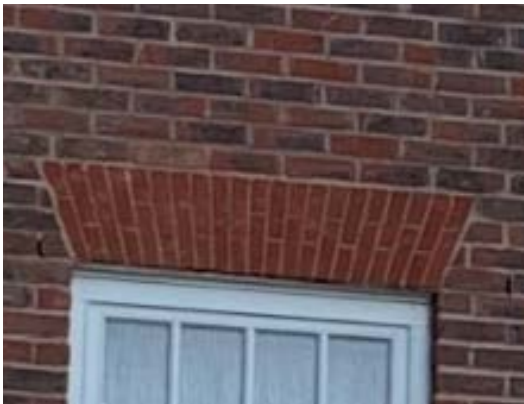
Flat segmental red brick arches
