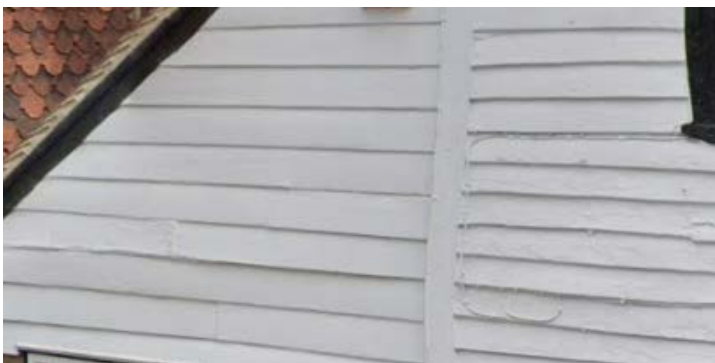
Differences between modern and traditional weatherboarding
