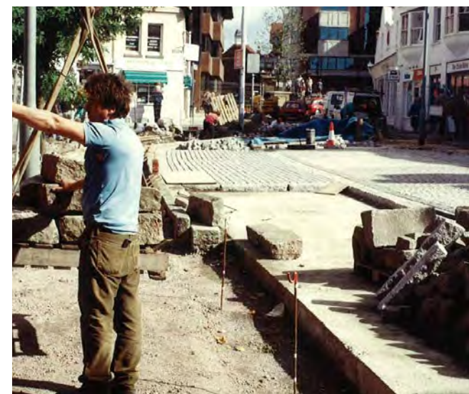
Granite setts originally being laid in the carfax carriageway
