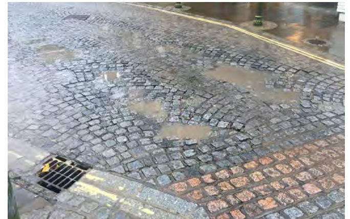
Existing setts in the carfax carriageway
