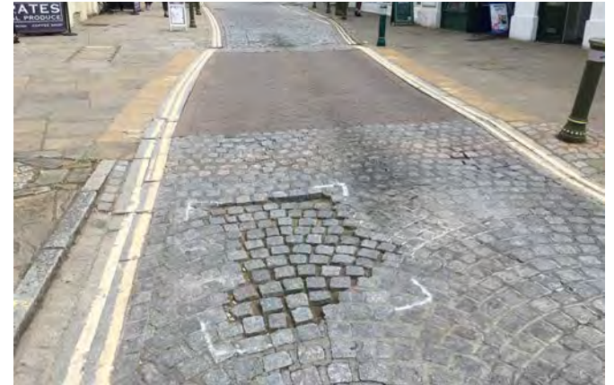
Existing setts in the carfax carriageway
