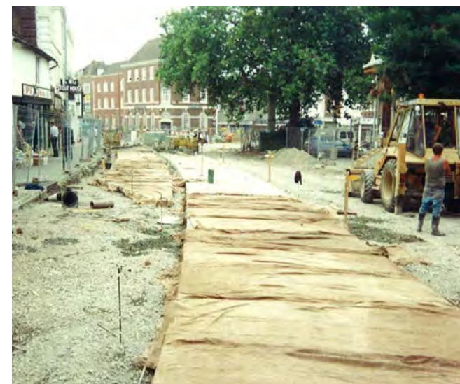
Granite setts originally being laid in the carfax carriageway
