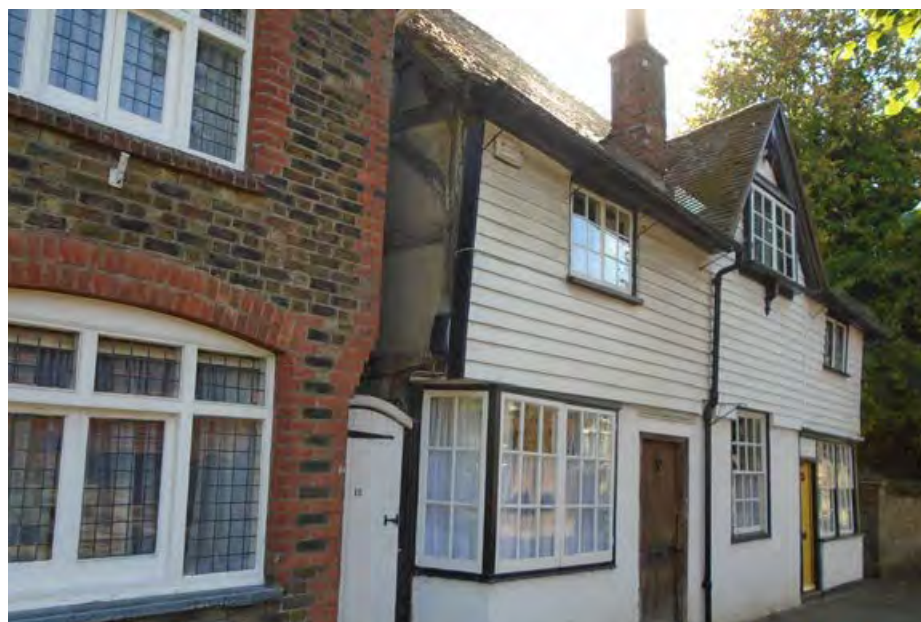
Timber frame set behind a weatherboarded frontage on Causeway
