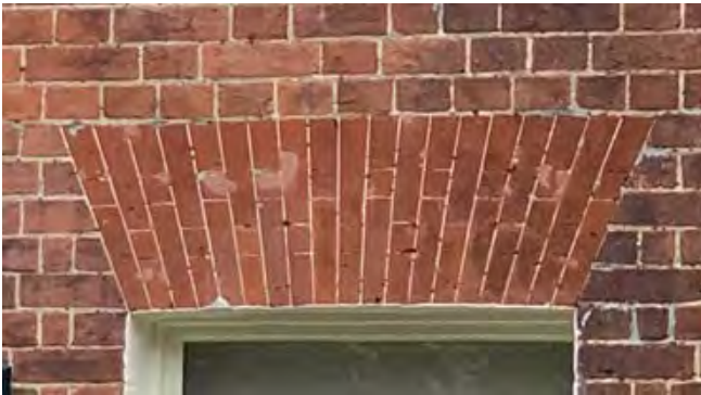
Flat segmental red brick arches
