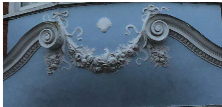
Decorative pilaster and cornice details
