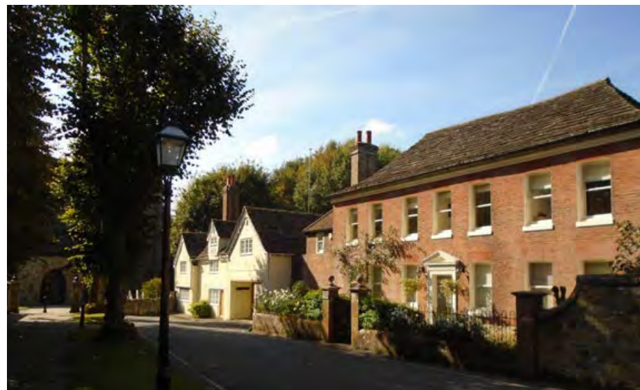
Horsham Stone Slate roofs within Causeway
