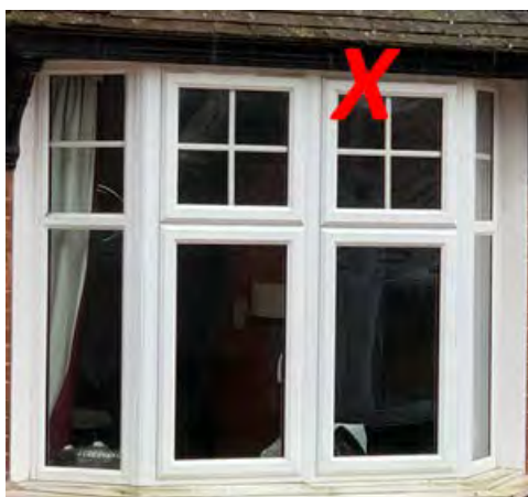
The use of plastic windows do not reflect the character of the conservation area, this is particularly evident in the lack of detailing and the changes to opening mechanisms.
