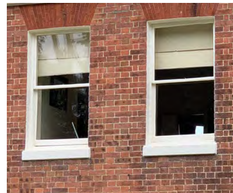
Positive windows within the conservation area showing historic sash windows, and in the image to the right historic glass with its distortions.
