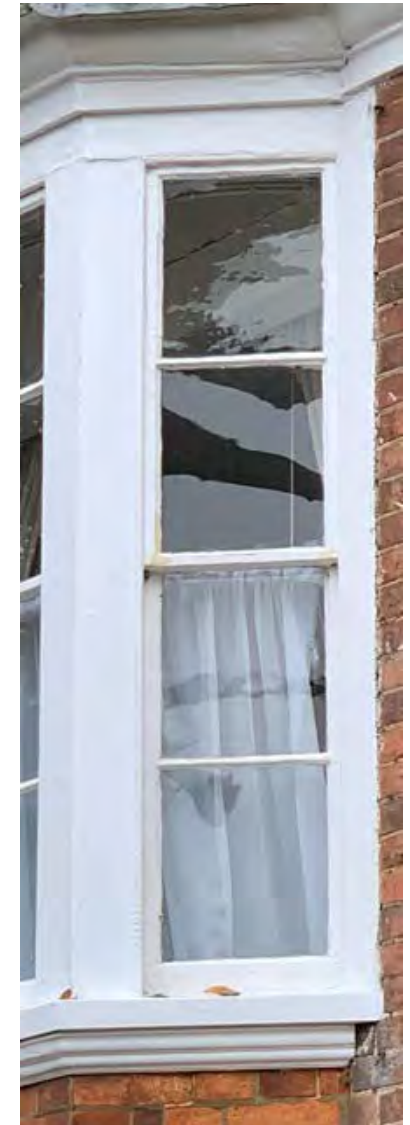
Positive windows within the conservation area showing historic sash windows, and in the image to the right historic glass with its distortions.
