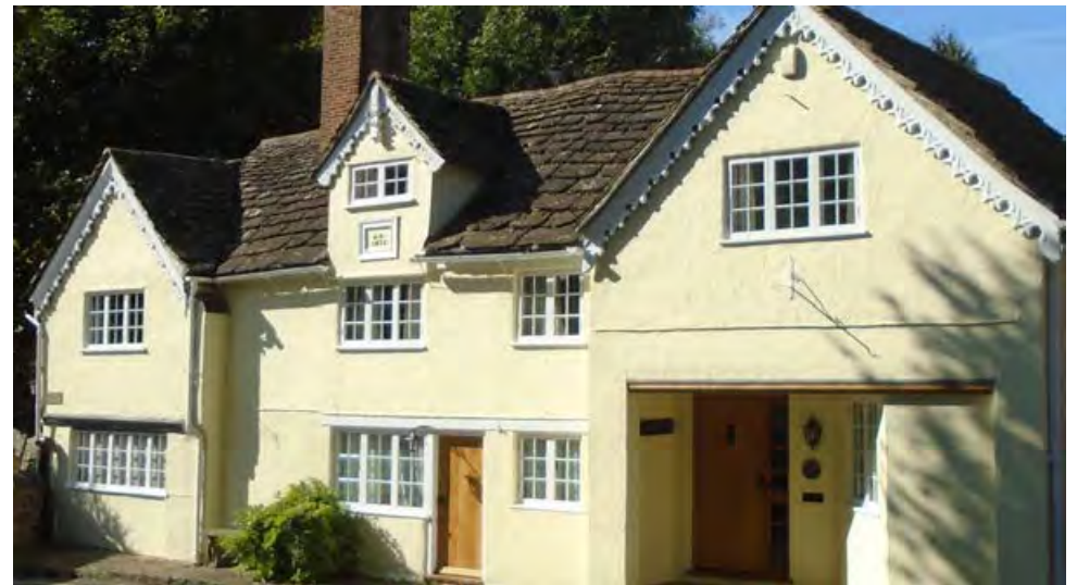
Horsham Stone slate roof
