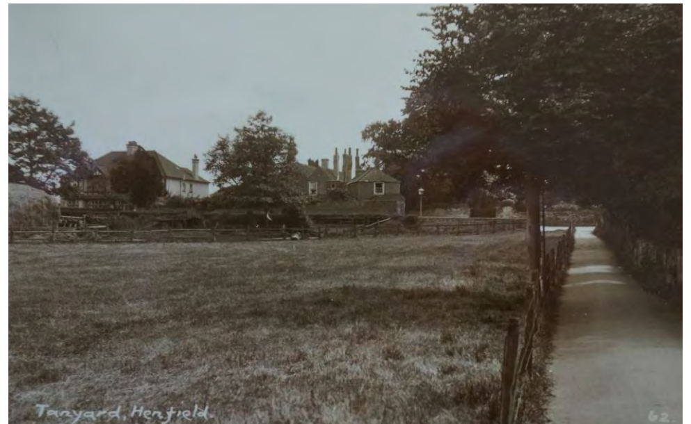
Tanyard, looking south towards Seven Chimneys.
