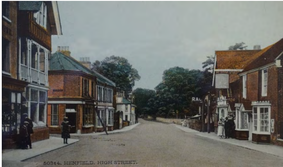
High Street, looking north.
