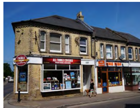
Turn of the century commercial buildings on the High Street
