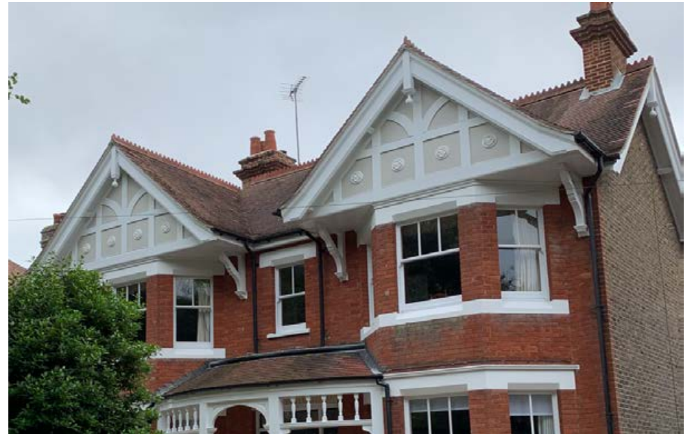
Timber sliding sash windows
