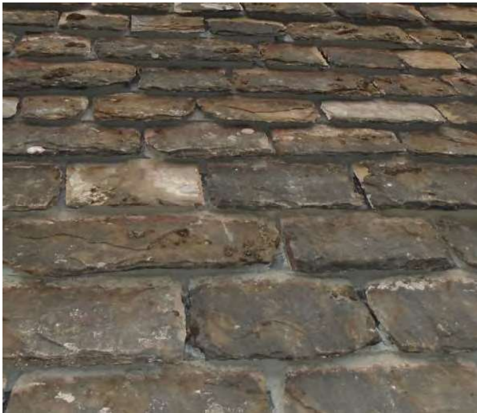
Laying of Horsham Stone slate roof with shadow slates and inconspicuous mortar
