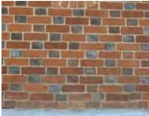
Flemish bond with dark grey burnt headers alternate header and stretchers
