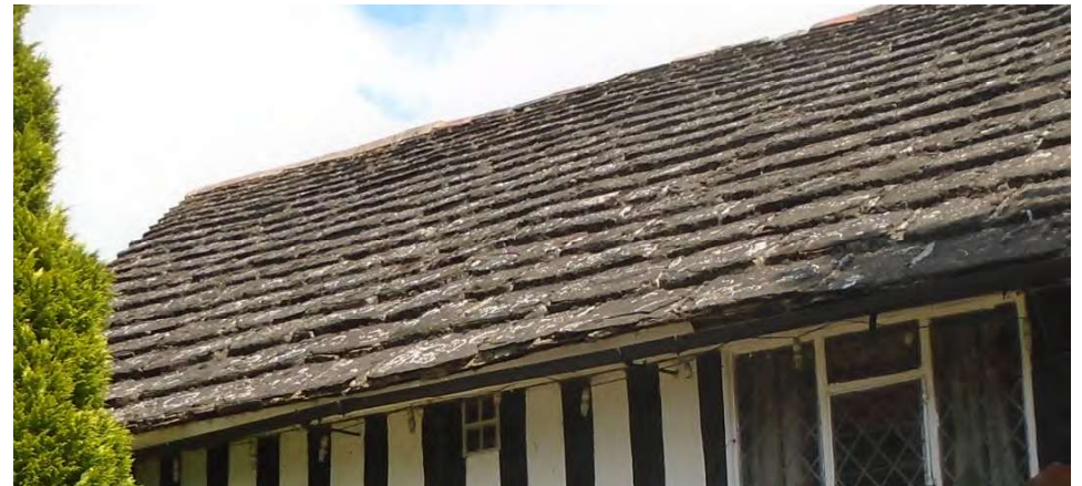
Horsham Stone slate roof
