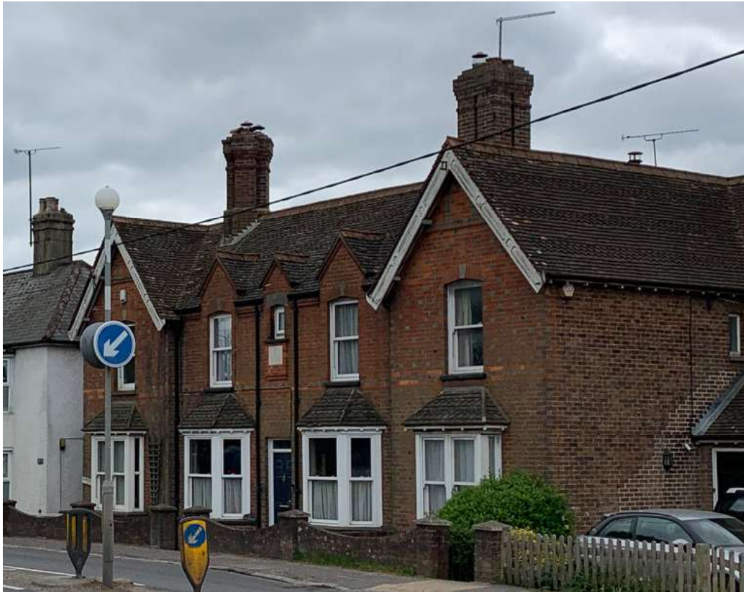
Bargeboards and finials ridge details and decorative roof tiling
