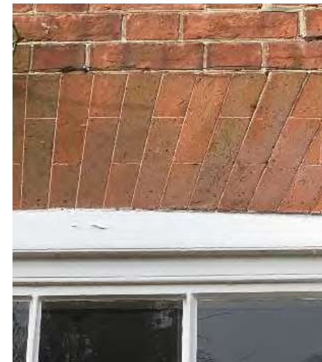
Decorative headers above the windows
