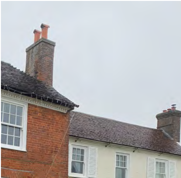
Examples of chimneys
