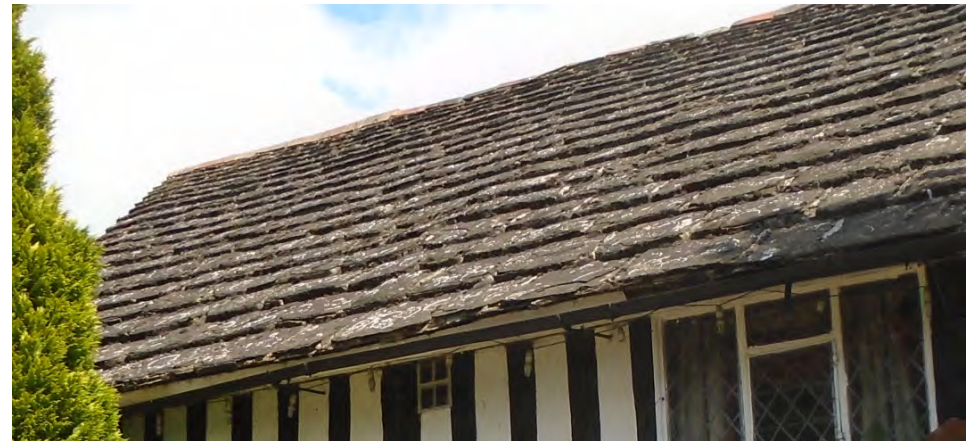
Horsham Stone slate roof
