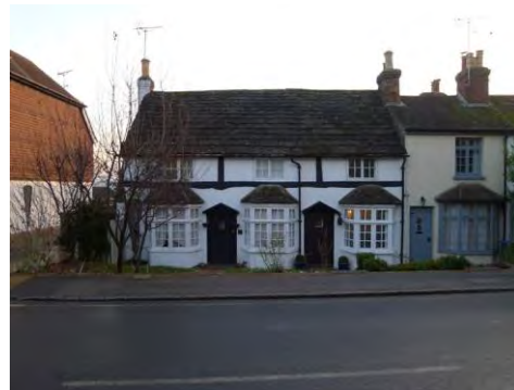
Horsham slate roofing
