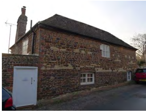
Carstone / Ironstone walling
