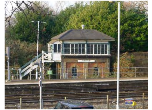
Listed signal box
