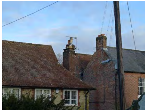
Characteristic roof forms and flank walls
